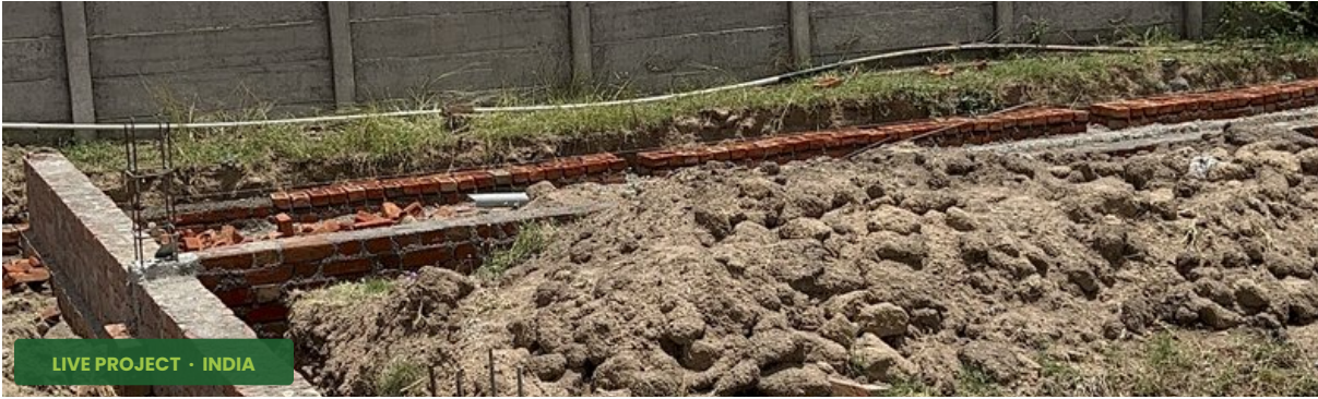
PLINTH & BOUNDARY WORK, PROJECT SITE
